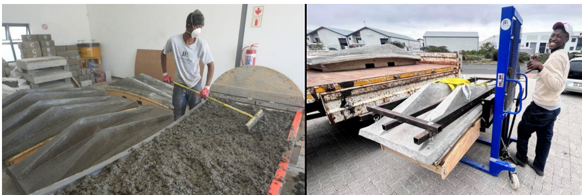
Figure 4. The funicular floors manufactured in halves and transported to site for assembly and finishing.
