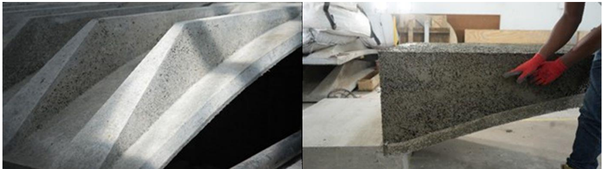
Figure 3. Rib-stiffened shell of structural mix (left) and non-structural in-fill creating walkable surface (right).
